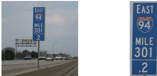
Figure 2 - Enhanced Reference Marker Example: 1-94 EB at Mile Marker 301.2
